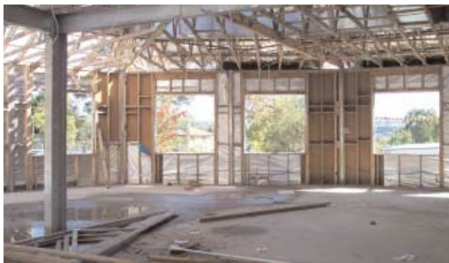
The Forestville Library and Community Arts Centre under construction.
