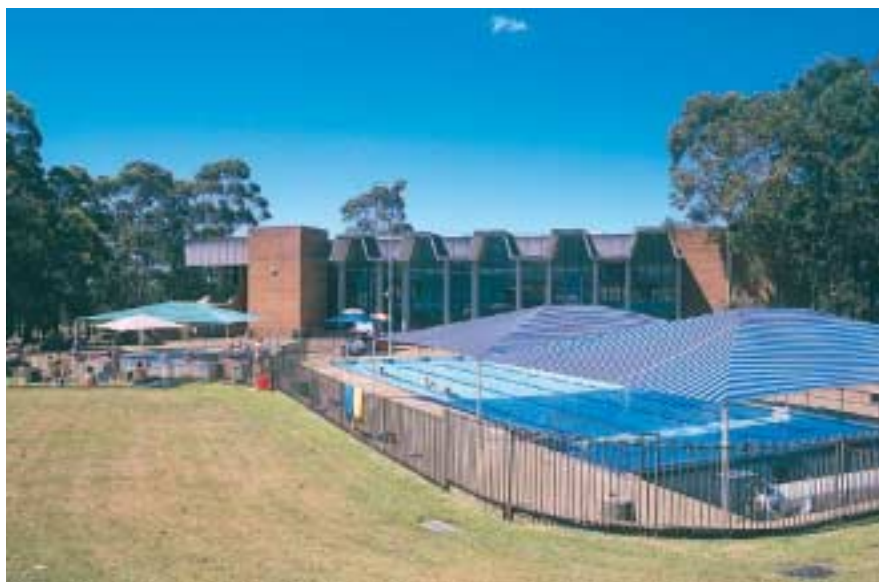
The outdoor pools at Warringah Aquatic Centre have been equipped with energy saving technologies.
