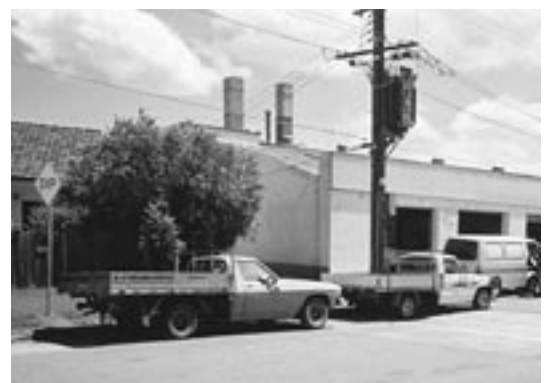
Air exhaust and stacks which have been constructed to consider the potential impacts on neighbouring premises.
