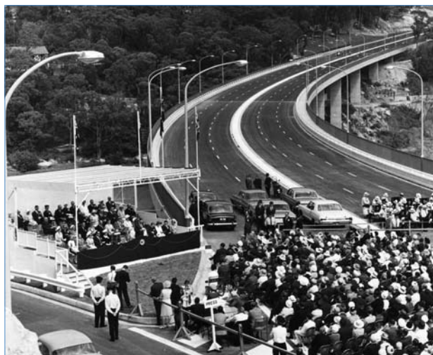
Roseville Bridge Opening in 1966
