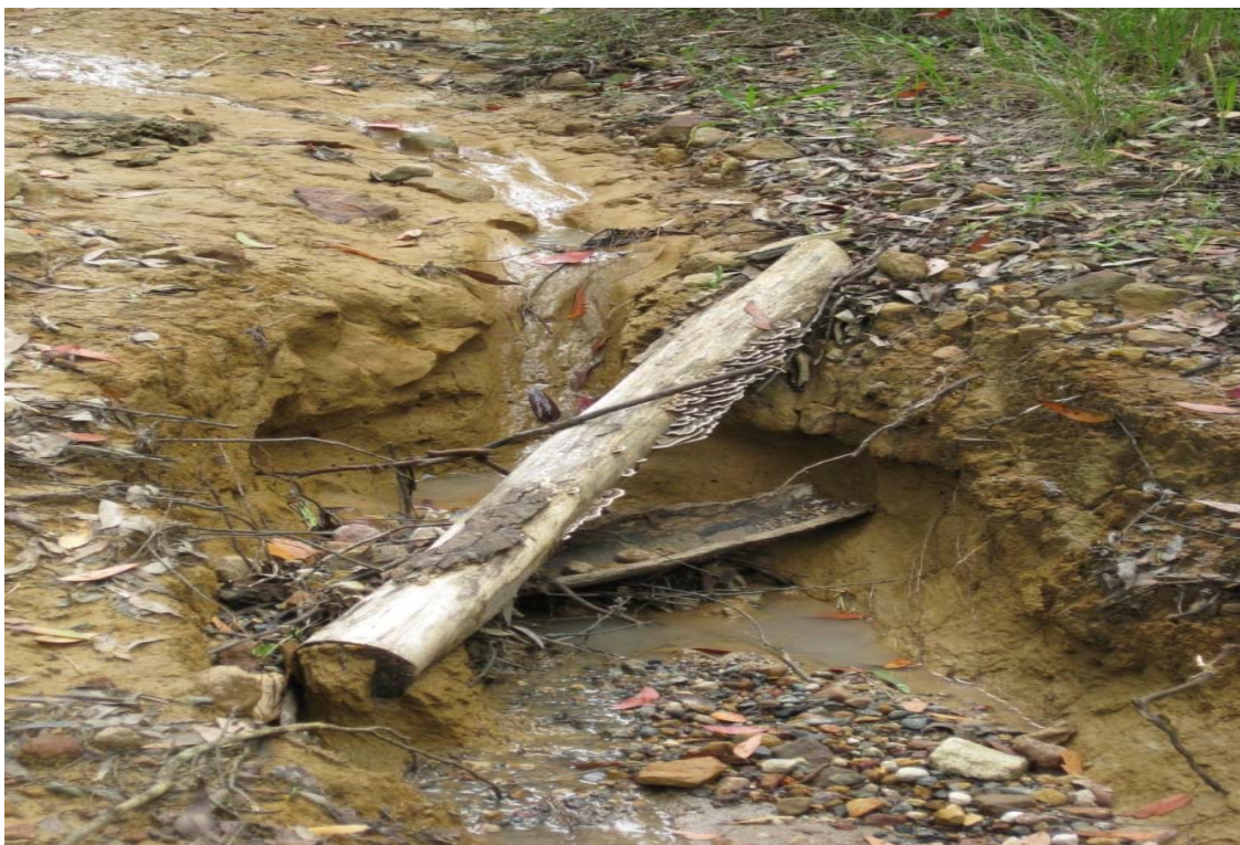
Erosion along the trail in Weemala Road (Unformed Crown Road)
